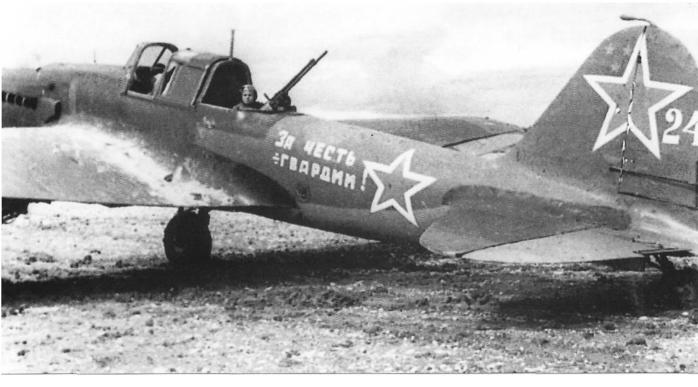
A Pictured immediately prior to take-off, this Ilyushin Il-2m3 shows very clearly the reargunner introduced with this model. The Red Air Force rarely tallied "kills" but the three stars on the tailplane indicate three victories, probably ground-attack targets. The writing on the fuselage indicates that this aircraft is part of a Guards formation.
