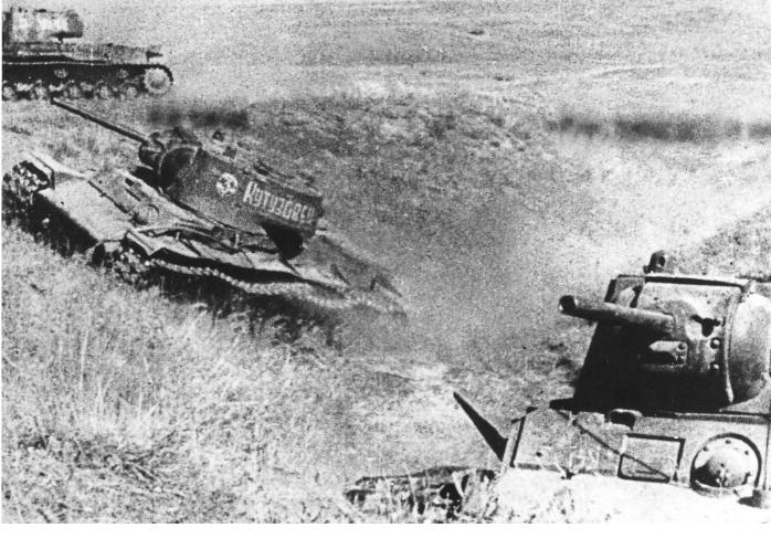
▲ Soviet KV-1 heavy tanks. At the beginning of the war against Germany the Red Army possessed 639 KV-1s. Armed with a 76.2mm main gun, the KV-1 could knock out all but the heaviest German tanks. However, because of mechanical problems, it was unreliable.
