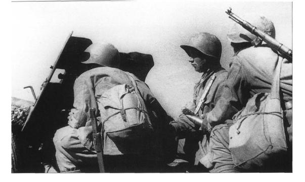
▲ Panzer front! A 45mm Model 37 antitank gun makes ready to fire. This gun was a derivative of the German 37mm antitank piece. The Soviets had increased the calibre to take larger, high-explosive shells to enable it to be used as an infantry support weapon. A new version, the Model 1942, was introduced before Operation Citadel.
